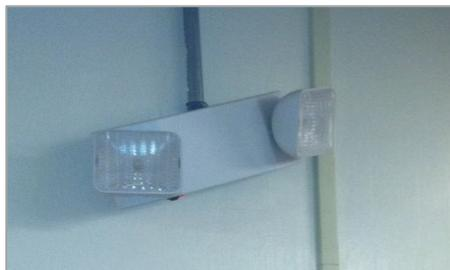
Make sure lights are intact and secured to the wall. This light is not properly connected.
